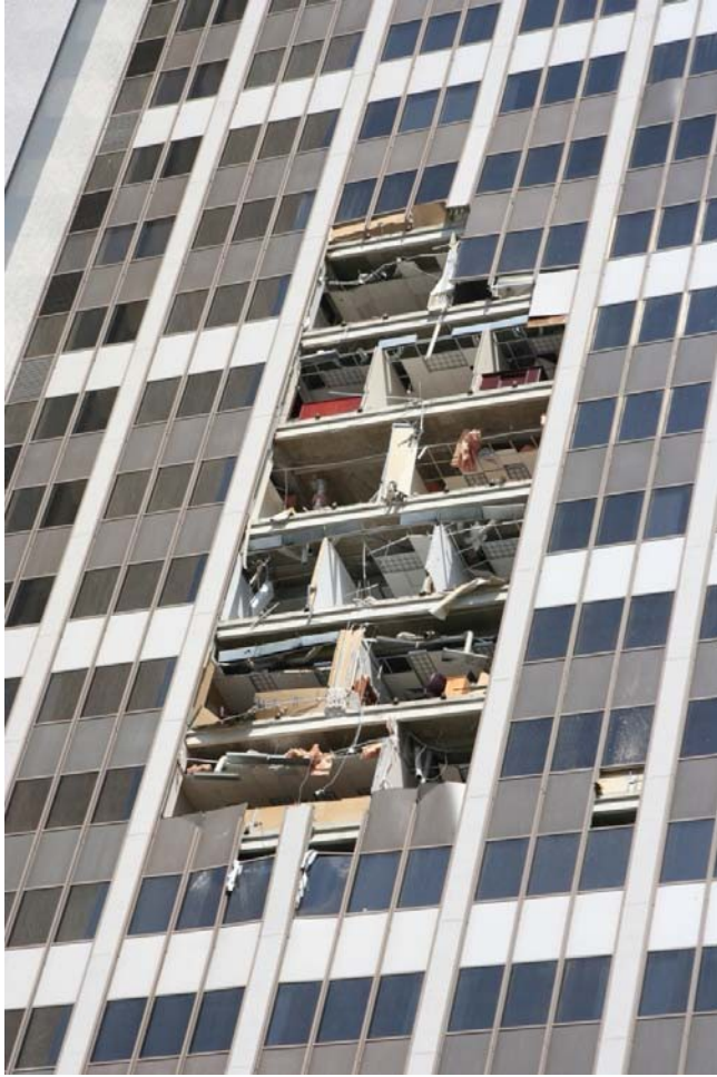
Figure 12. Exterior photograph of exterior wall. A spectacular, catastrophic collapse resulting from uncoordinated support of a curtain wall.. Jamb aluminum mullions were exclusively supported onto adjacent CMU piers, which had insufficient load resistance to collect design reactions from the curtain wall. Photo credit – Mr. Alessandro Abate.
