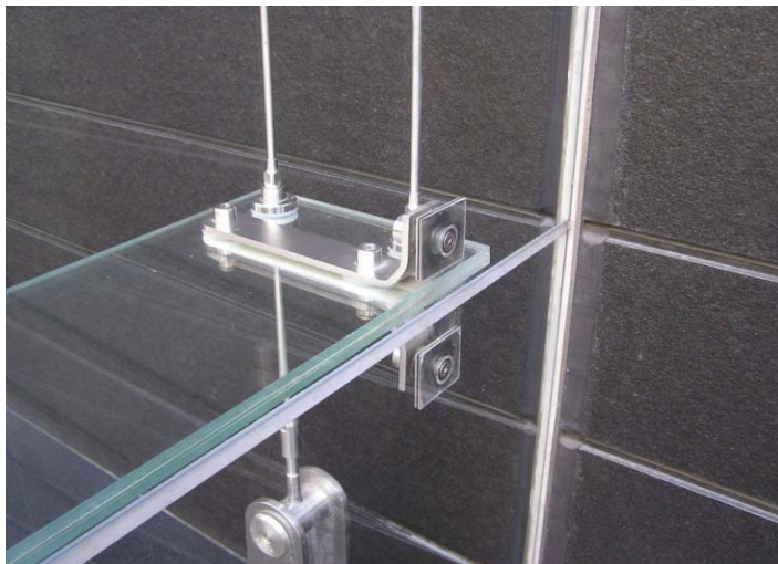
Figure 1. Example of the vocabulary challenge. The structural glass wall, with horizontal structural glass mullions suspended on stainless steel cables. The glass fins play structural role by resisting lateral load, as opposed to the traditional load-collecting role of glass. No structural sealant used here.
